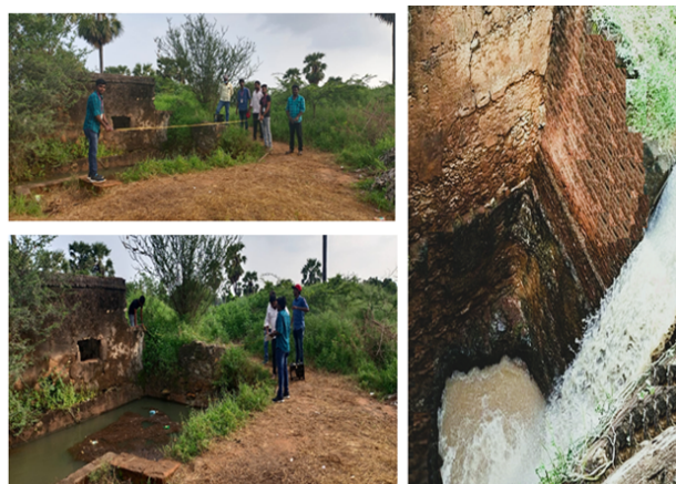
Figure 3: Artificial Recharge System at Ayyankulam Well.
