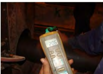
Figure 7: Pipe temperature before epoxy application.
